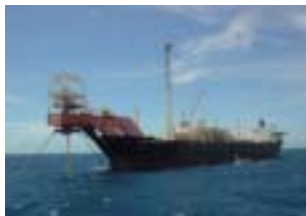
PEARL Jasmine FPSO (Thailand)
