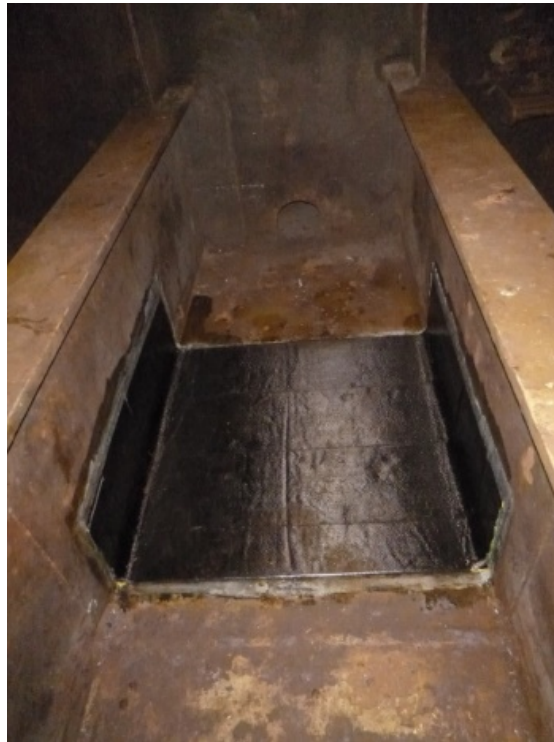
Repair of Bottom Plate by using CFRP
